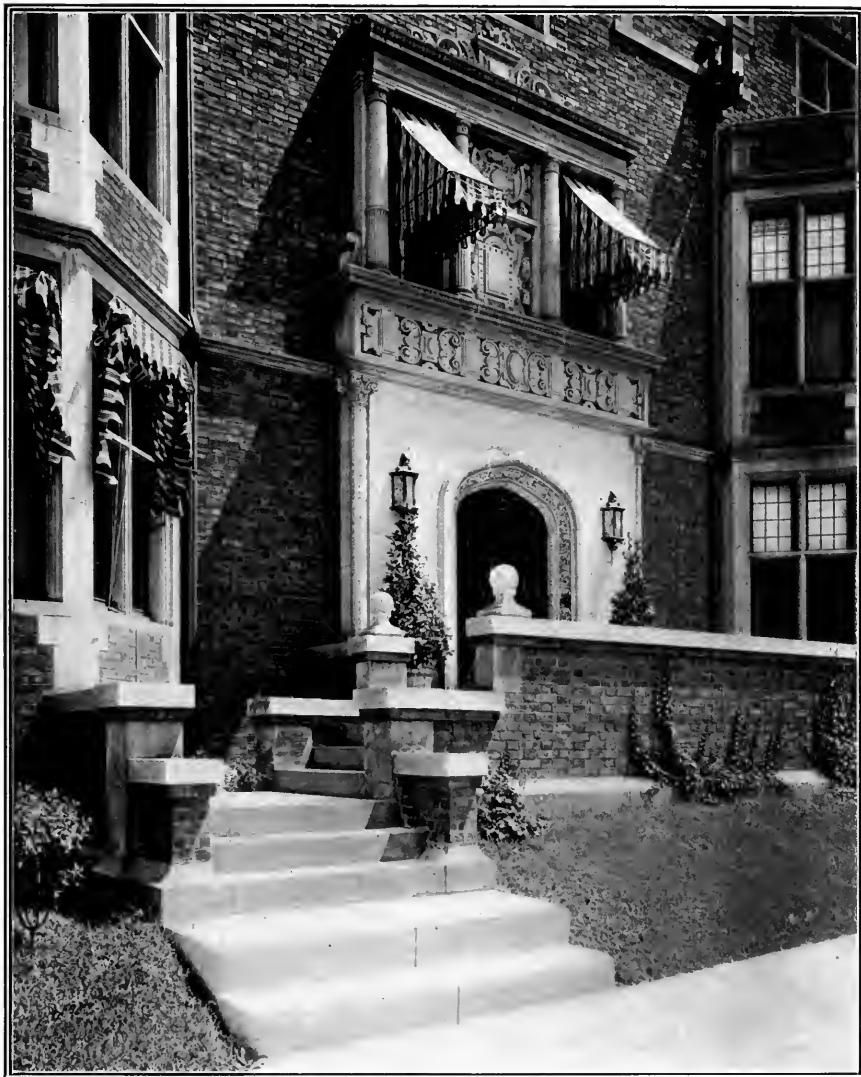
ENTRANCE OF BLACK RESIDENCE.
